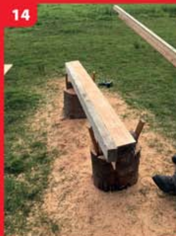
14 Extension piece in position.
