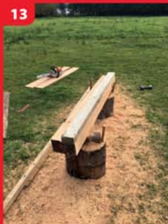
13 Fitting extension piece to cut last boards.
