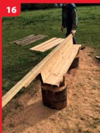
16 Last boards cut.
